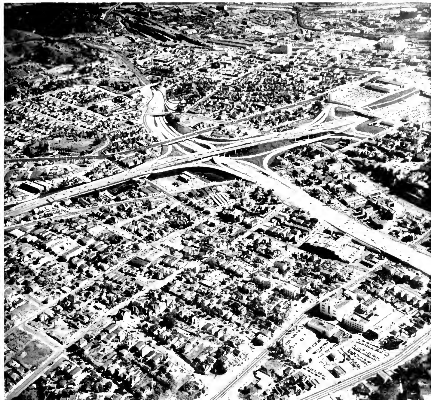
Looking northeasterly, showing four-level traffic interchange in center of photograph; Hollywood Freeway extending from center left to upper right, and Harbor Freeway and Arroyo Seco Freeway extending from lower right to upper left
